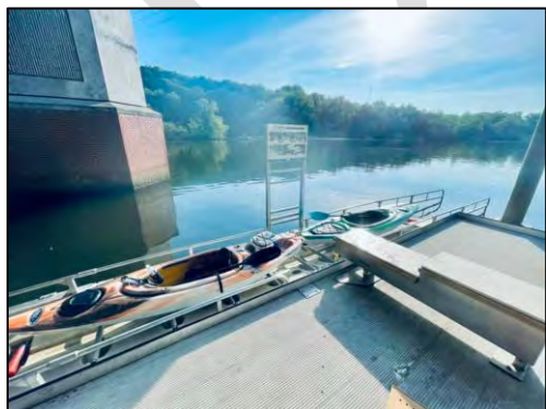
Figure 11 Kayak Launch Ramp completed, 2021
