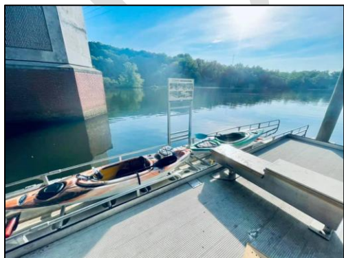
Figure 11 Kayak Launch Ramp completed, 2021
