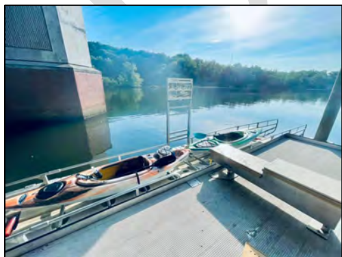
Figure 11 Kayak Launch Ramp completed, 2021
