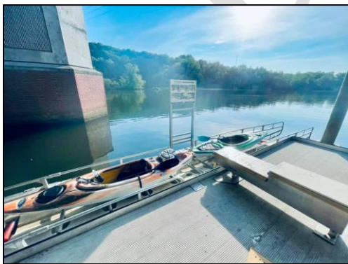
Figure 11 Kayak Launch Ramp completed, 2021
