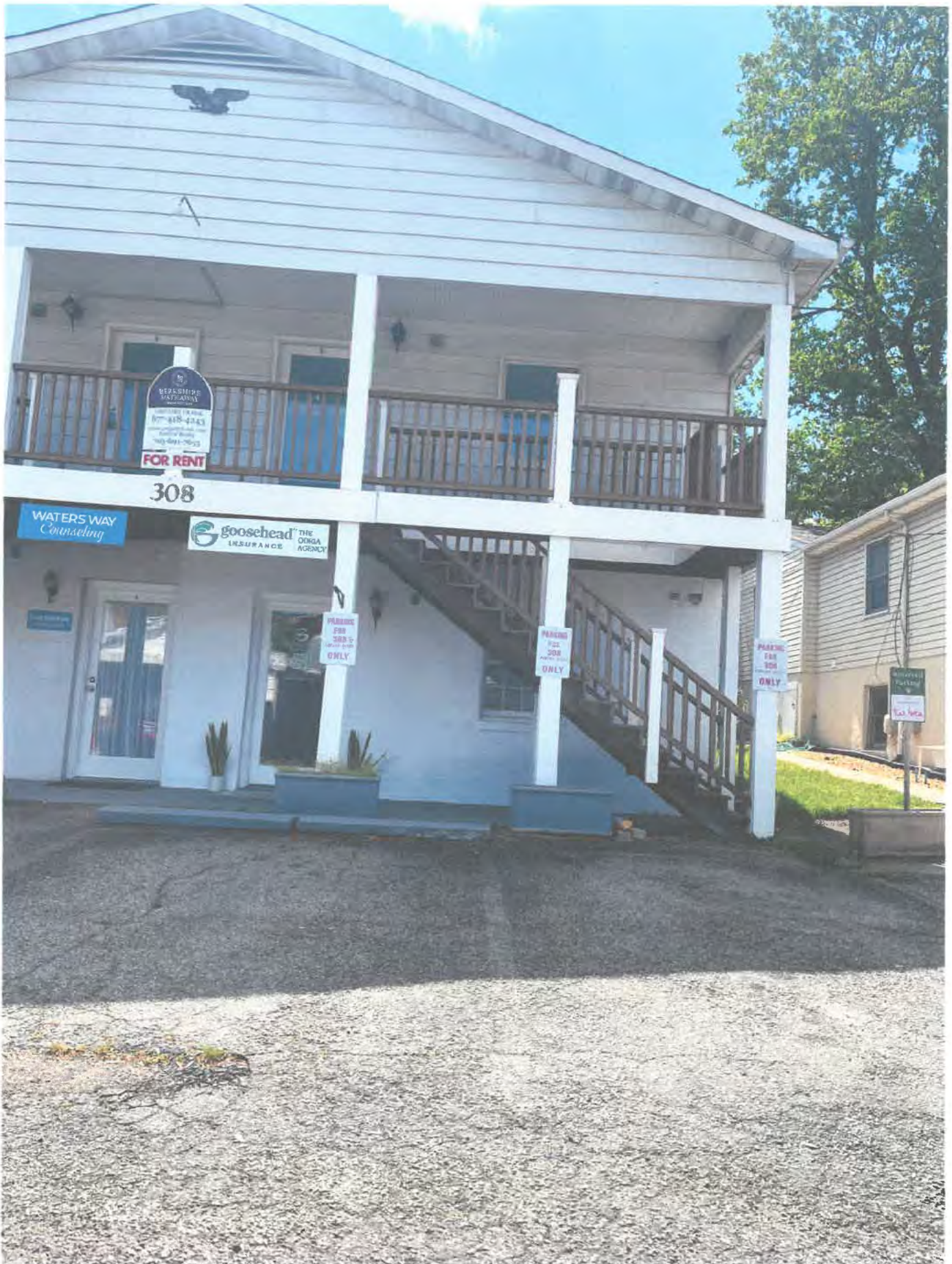
Backside 308 Boehr Alley re asphaltting parking area
