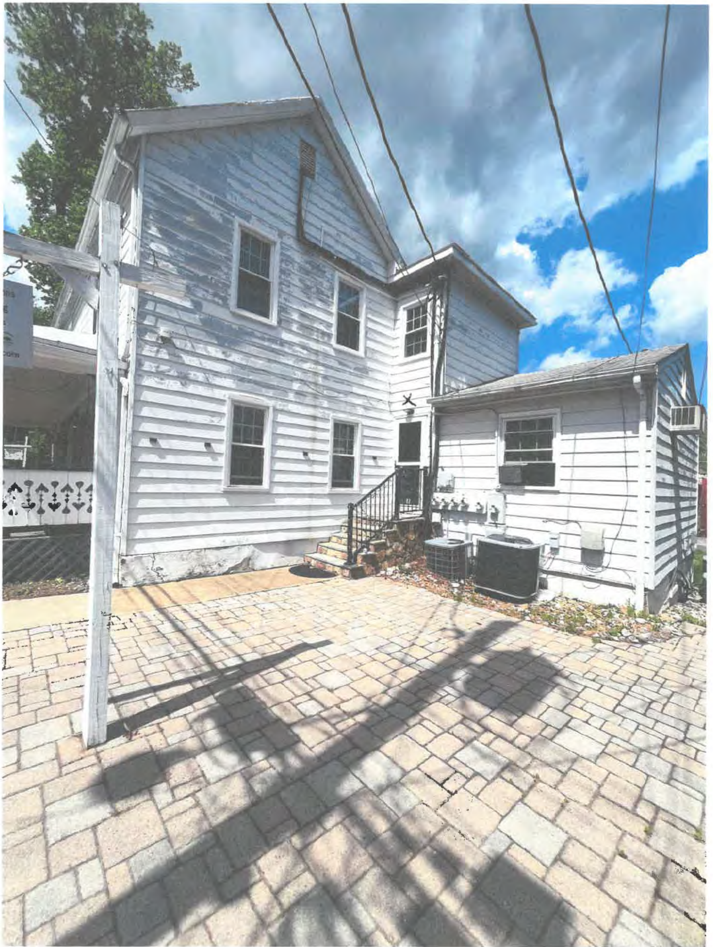
Side of 303 Commerce St. Proposed shed roof over door
