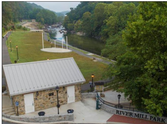
Figure 6 Former site of Water Treatment Facility, River Mill Park completed in 2016
