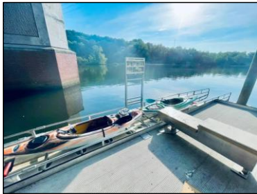
Figure 11 Kayak Launch Ramp completed, 2021
