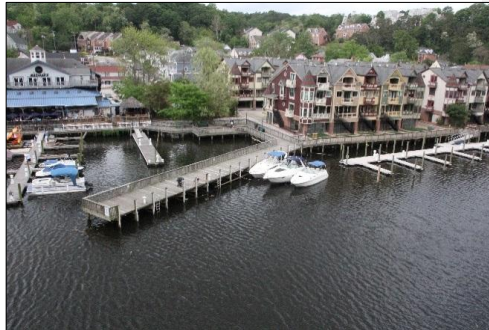
Figure 8 View of Riverwalk and Town Dock, 2015
