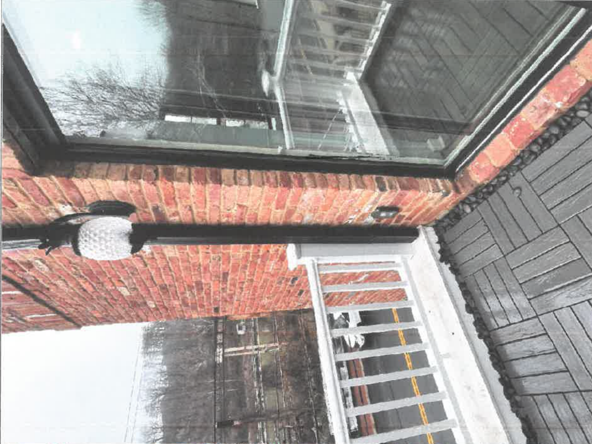
Old PVC railing that is not up to code
